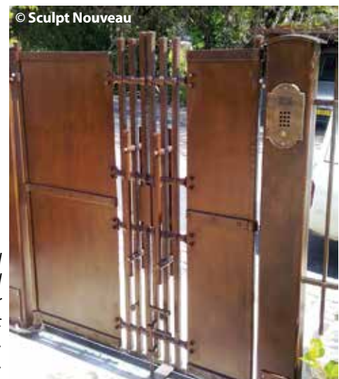
Japanese Brown applied cold on cold rolled steel. Sealed with Ever Clear two part acrylic urethane clear coat. Patina by Israel Garcia.
